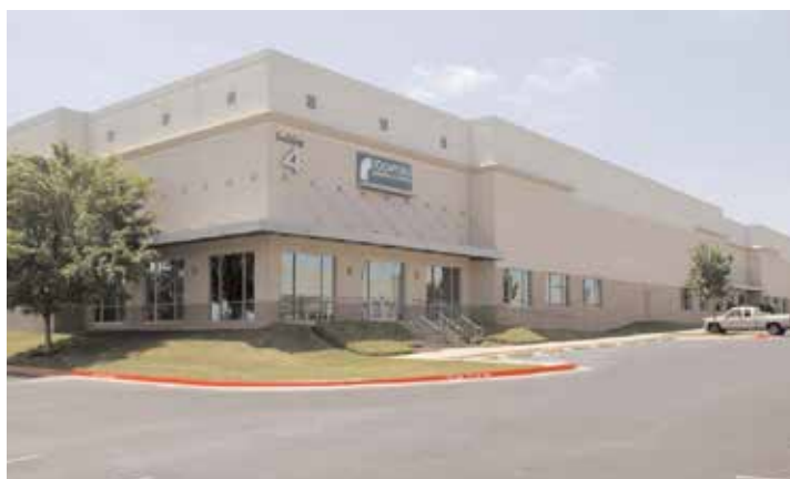
South Park Commerce, Austin, TX Industrial
